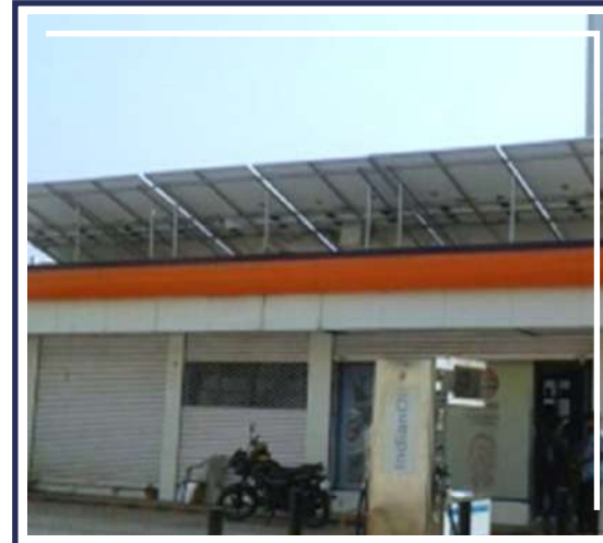
Experience of Solarizing, 400+ Petrol Pumps of IOCL and HPCL Across INDIA
